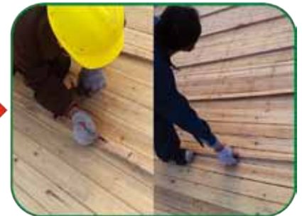
Do a horizontal line and test to check for level materials
