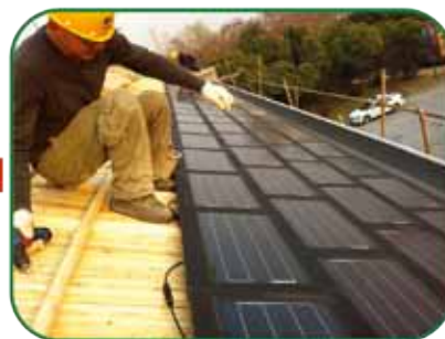
The photovoltaic tile roof is completed
