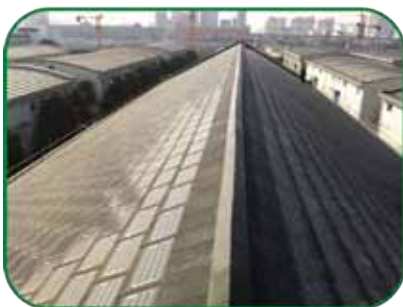
Install the counter batten and roof batten
